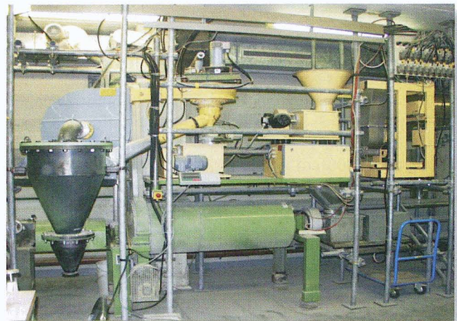
Figure 3: Semi-industrial ball mill at the Research Institute of the Cement Industry
